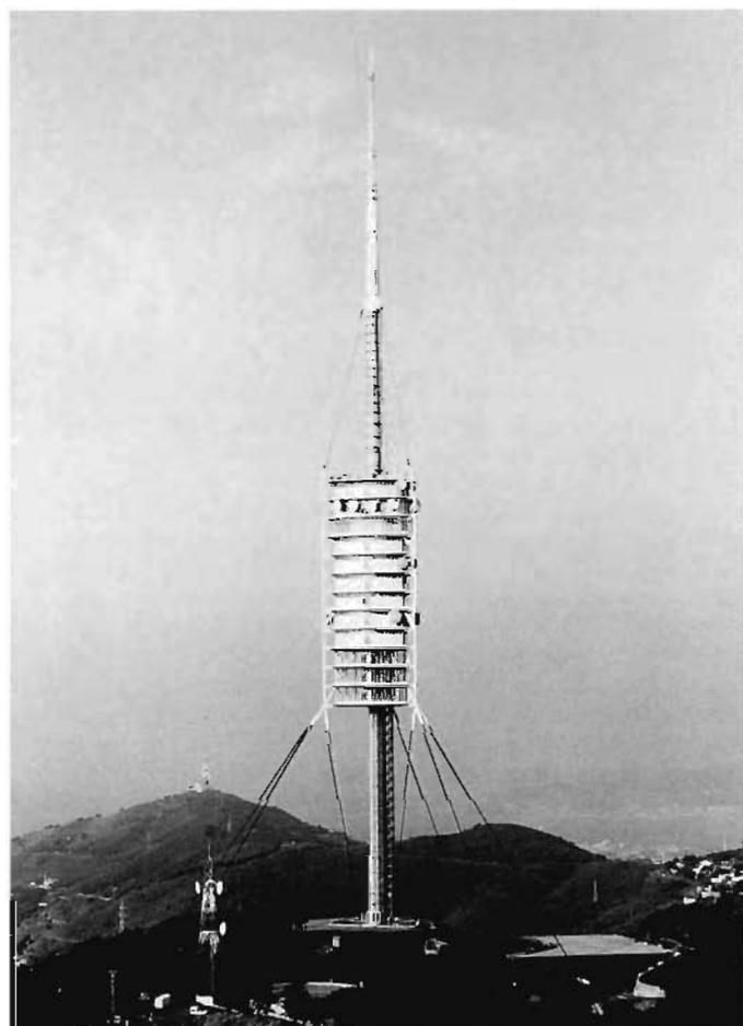
connections have been used, with long radius internal curves to minimise local stress concentrations. Full-scale prototype testing of the guys and their connections was carried out by the manufacturer, Verto Phyllystran of Holland.
